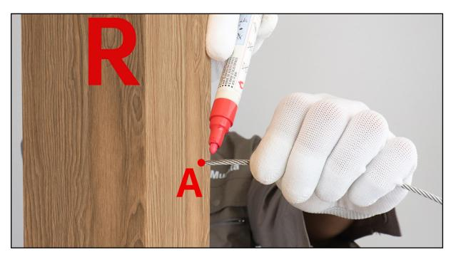
**Step 6 -** Tighten the cable **5** from the right end post, mark point A from the outside, and cut cable on point A with cable cutter **6**.
