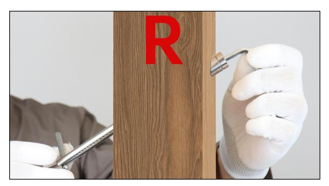
**Step 9 -** Put in angle washer **3**, and tighten the tensioner **1** with an Allen wrench **4** and socket wrench **1** on the right end post.
