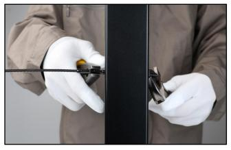
**Step 3 -** Crimp the tensioner with cable and install the tensioner. Tighten the cable with wrench to achieve the required tension.
