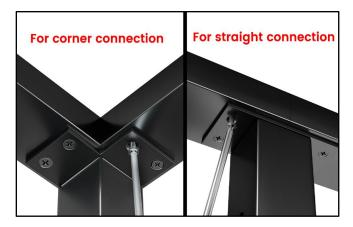
Step 2 \_ Drill the holes, connect the handrail and bracket (for with screws metal **6** (for handrails) or wood handrails).
