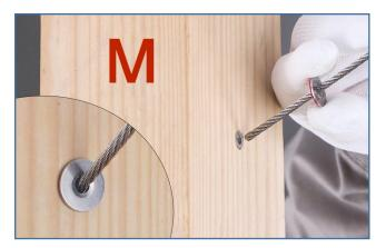
**Step 3 -** Pass cable **6** through all adhesive washer **10** and intermediate posts.
