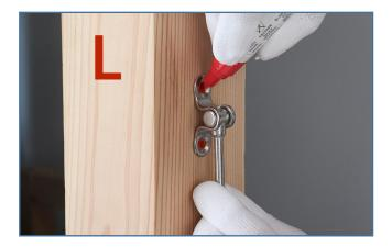
**Step 4 -** Locate fixed end **2** on the left end post, mark holes.
