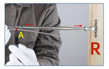
**Step 9 -** Pull the cable straight, mark the cable at the flatten part (point A) and cut at point A with cutter 7.
