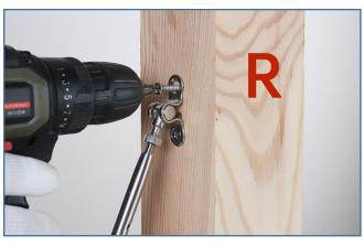
**Step 7 -** Use screws **3** to fix tensioner **1** on the right end post.
