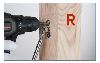
Step 8 - Use screws ③ to fix tensioner ① on the right end post.
