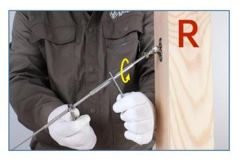
Step 12 - Clamp tensioner ① with a plier, use bent wrench ④ to tighten the cable.
