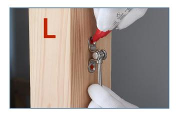
**Step 5 -** Locate fixed end **2** on the left end post, mark holes.
