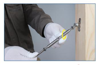
**Step 9 -** Loosen tensioner **1** to extend the turnbuckle to about 3/4.
