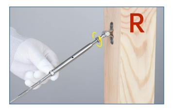
Step 13 - Fix tensioner **1** with two nuts to prevent it from loosening.
