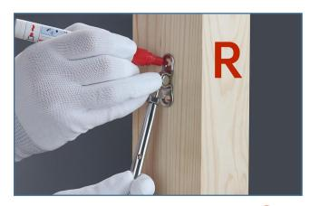
Step 7 - Locate tensioner 1 on the right end post, mark holes.
