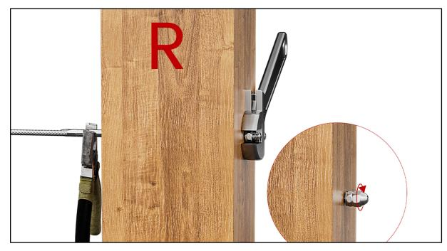
**Step 9 –** Install the tensioner **1** with clamp and wrench on the right post.
