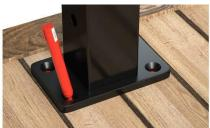
Step 3 - Place 4 on floor, mark 4 position in the holes of 1 with a pen.
