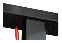
**Step 1** - Place the handrail above the bracket, mark the holes position on handrail.
