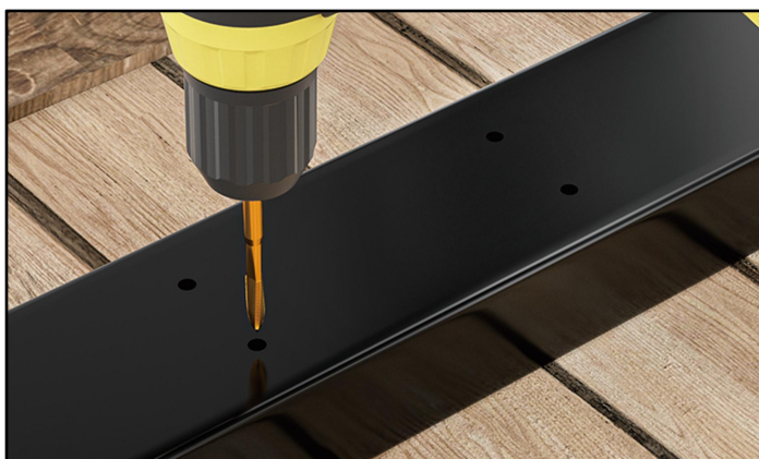
Step 3 - Drill threads using a M5 drill tap.
