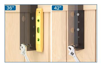
**Step 7 -** Use spirit level to make sure the post 1 is perpendicular to the ground. Then tighten the lag screws 9 with wrench.
