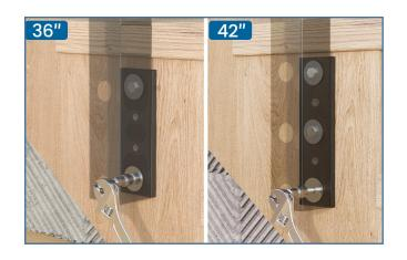
**Step 9 -** Use spirit level to make sure the post is perpendicular to the ground. Then tighten the lag screws **9** with wrench.
