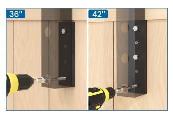
**Step 6** - Use electric drill with nut setter **6** to install M8 lag screws **9**. Leave them a little loose for final tightening.
