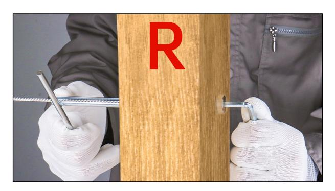
**Step 9 -** Tighten the tensioner **1** with the Allen wrench **1** and socket wrench **4** on the right post.
