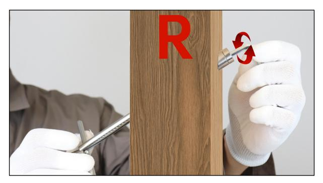
**Step 9 -** Install the angle washer , tighten the tensioner 0 with the Allen wrench 0 and socket wrench 0 on the right end post.
