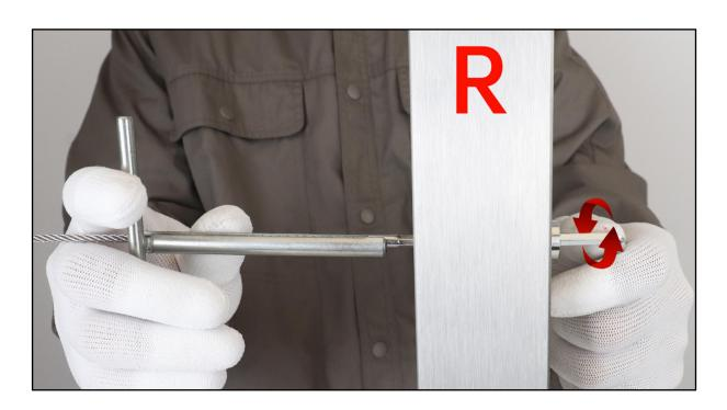
**Step 7 -** Tighten the tensioner ① with the Allen wrench ② and socket wrench ④ on the right end post.
