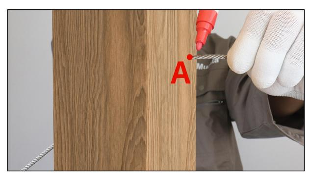
**Step 6 -** Pull the cable ② against the right end post, mark point A from the outside and cut cable ② on point A with cable cutter ③.
