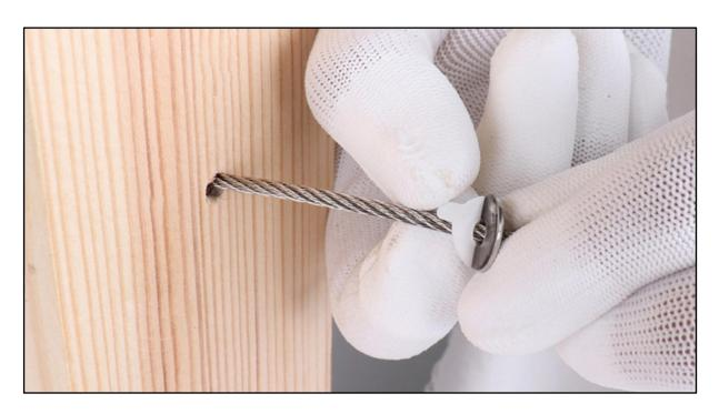
**Step 10 -** Install the adhesive washers **3** and level protector sleeves **5**.
