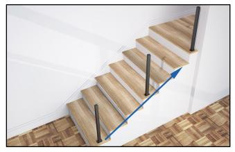
**Step 2 -** Draw a horizontal line to ensure that the posts **(1)** are aligned.
