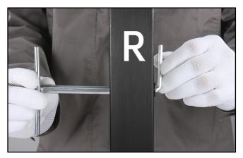
**Step 7 -** Tighten the tensioner with socket wrench 3 and 5mm Allen wrench on the right end post.
