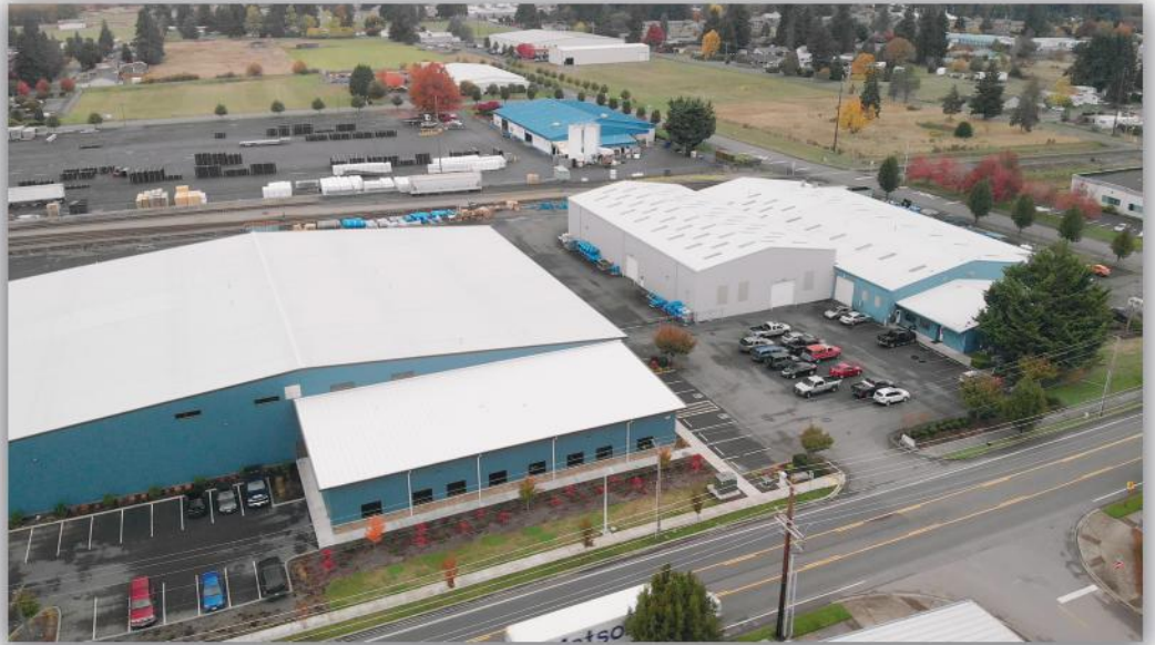
Centralia Branch Office, Production and Warehouse Facilities Centralia, WA
