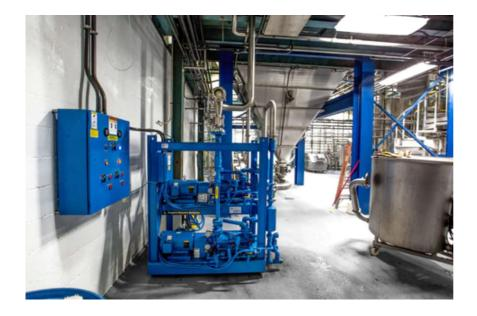
The Rogers Vacuum System selected by Organic Valley includes automatic loading controls which selectively operate and sequence the vacuum system pumps on and off based on actual demand, allowing for power and water savings. This system also includes the use of a soft starter to not overuse power when starting up.
