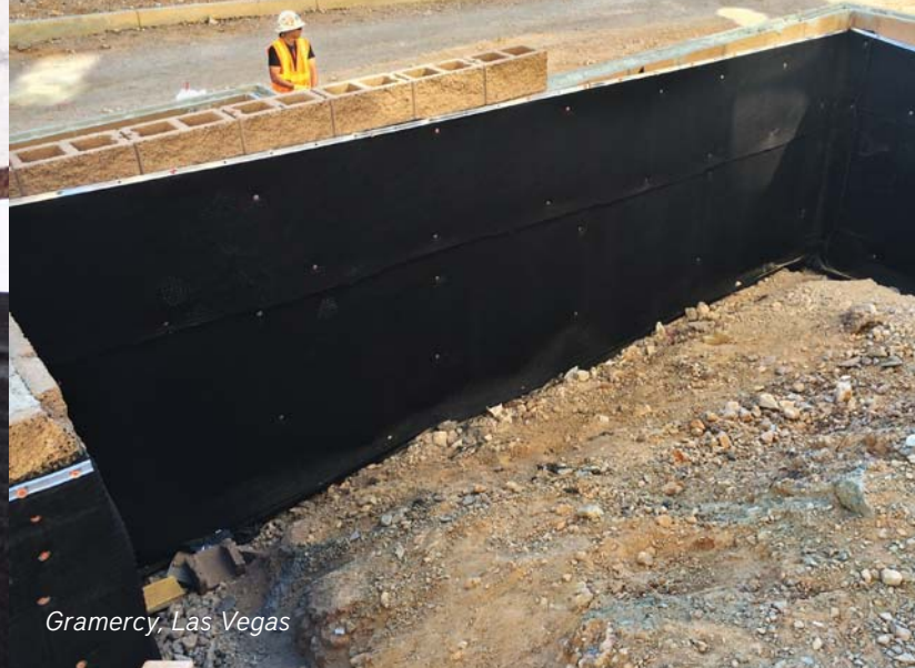
Central Region Elementary School #13 Parking Garage, Los Angeles
