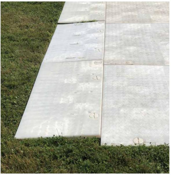
The first step is to lock male ramps in place along the entire length of the leading female edge of the panels.
