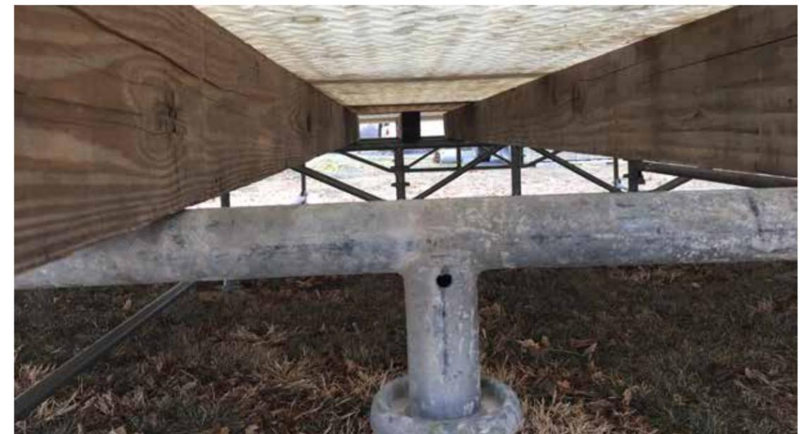
*Support beams should be positioned 22" apart so one beam rests under the center of the panel.*
