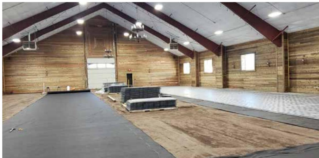
*A geotextile fabric covering can be installed first to create a barrier.*
