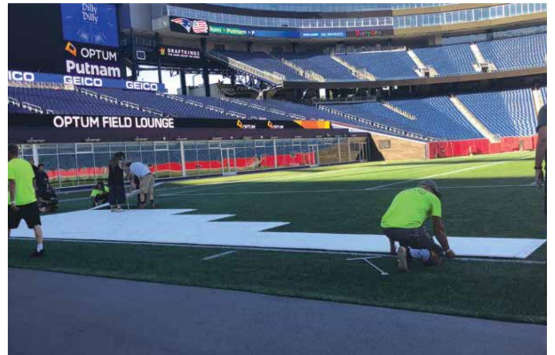
Check and recheck the alignment of the panels against the string lines to ensure panels stay straight.
