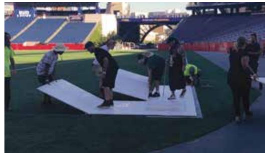
Lay the next pair of panels to extend the build in two directions.
