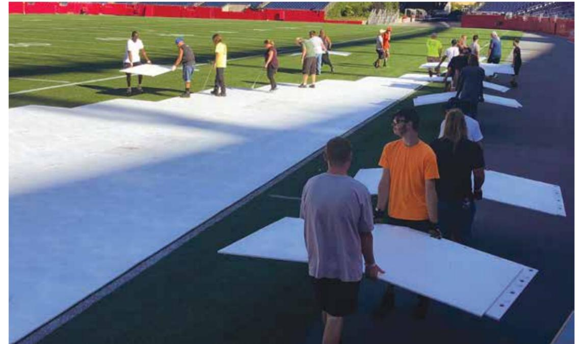
To avoid knocking panels out of alignment, keep installers and equipment off the panels until a substantial section of the flooring has been locked in place.
