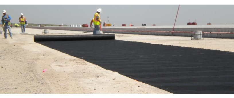
**GEOTEX® Nonwoven** geotextiles are made from the highest quality polypropylene staple fibers and needle-punched to form a dimensionally stable fiber network and include fabrics for separation and stabilization, subsurface drainage, filtration, and cushioning. This family of nonwoven products offers proven performance, is compliant with AASHTO/NTPEP standards, and is available in a variety of styles to fit your specific project needs and specifications.
