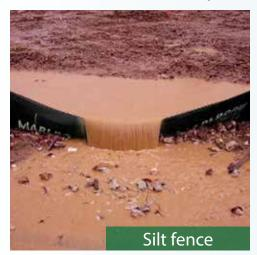
The sediment removal shortcomings of silt fence need little explanation. Failures such as this require regular maintenance, contributing to a much higher overall project cost.
