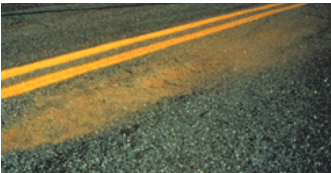
Figure 1 - Subgrade pumping
