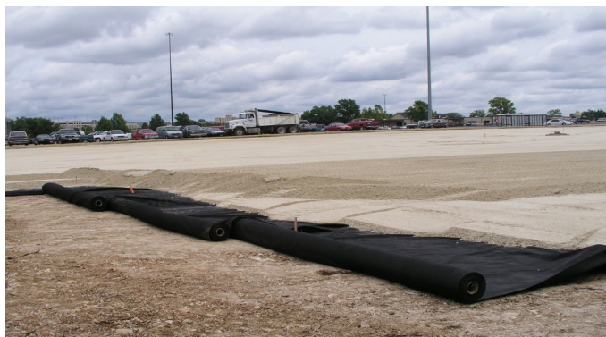
Figure 15 - Nonwoven deployed on subgrade
