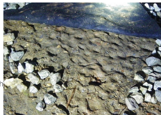
Figure 12 - Rock interlock on subgrade - excellent aggregate confinement with nonwovens
