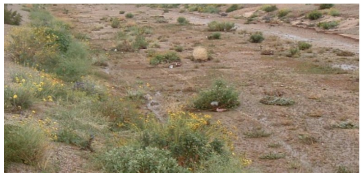
SOLUTION PYRAMAT® 75 was used to line the refurbished channel
