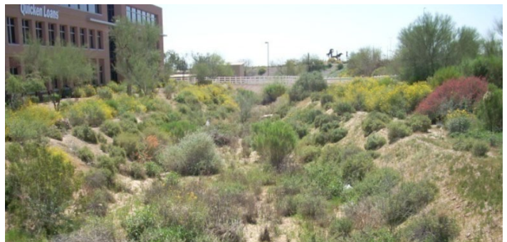
PERFORMANCE Aesthetic hard armor alternative with native plantings
