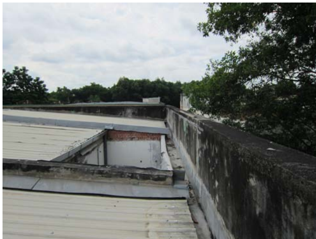
Trees located too near to the bird house will obstruct swiftlets' flight path and encourage intrusion of predators.
