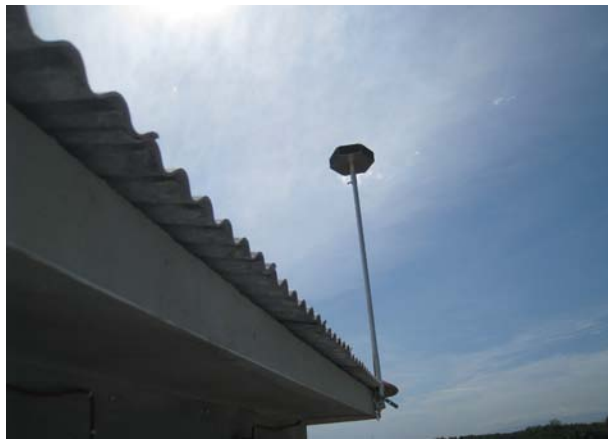
Installation of the hexagonal sound tweeter.
