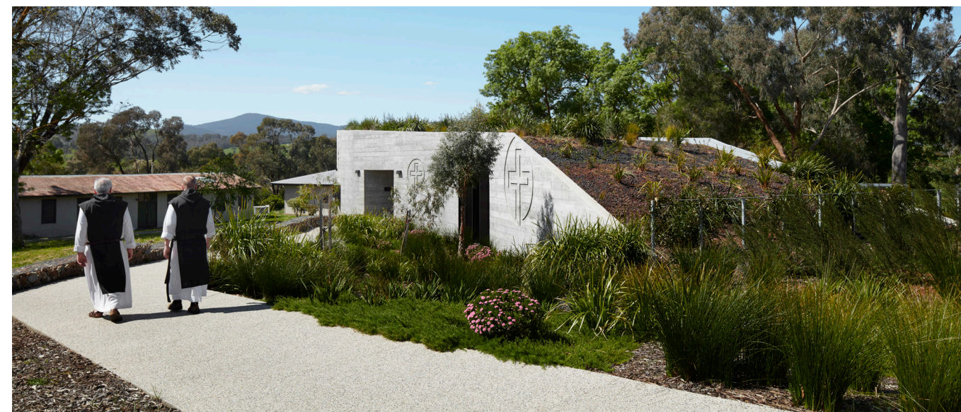
Above and right: Baldasso Cortese Architects, Tarrawarra Abbey , 2016. Photo: Peter Clarke, Latitude.
