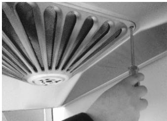
Align the Phillips screwdriver with the screw hole and raise it upward forcibly meanwhile rotating it counter-clockwise about  $120^\circ$ , so as to remove the screw out of the cross slot of the exhaust fume collecting hood.
