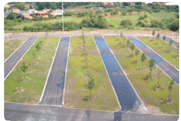
Gravel Cell® reinforcement structure used for access roads. Turf Cell® reinforcement structure used for parking bays.
