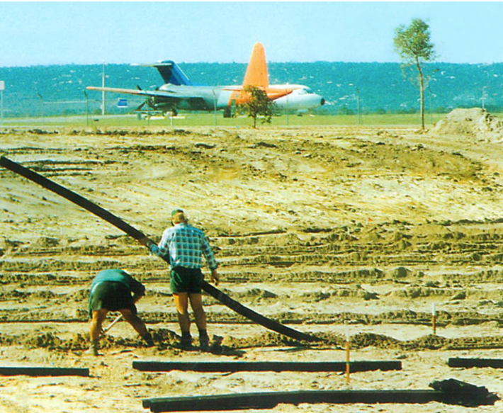
Perth Airport, Perth WA.
