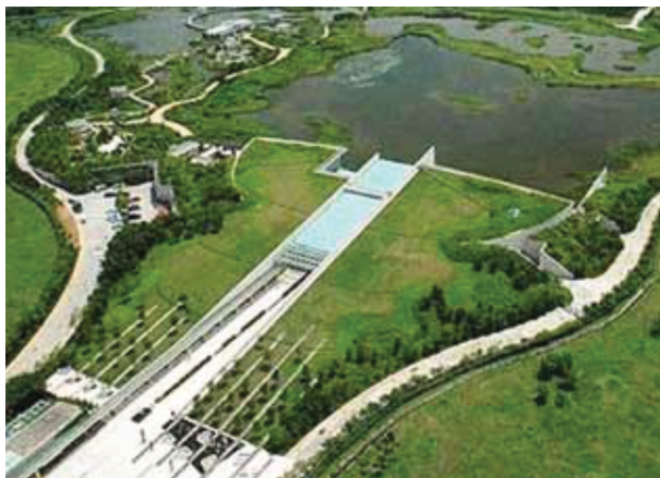
Installation in Hong Kong Wetland Park
