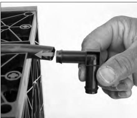
10. Complete installation of the remaining irrigation connections.
