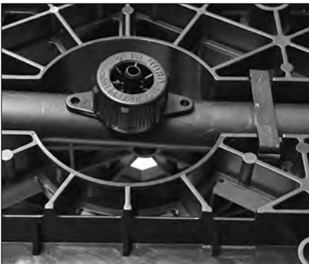
7. Install Drip Emitter through out the installation.
