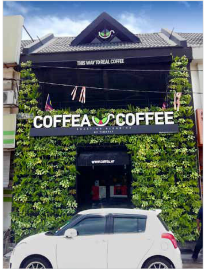
Gro-Wall® 4 installed onto coffee shop frontage in Kuala Lumpur, Malaysia.
