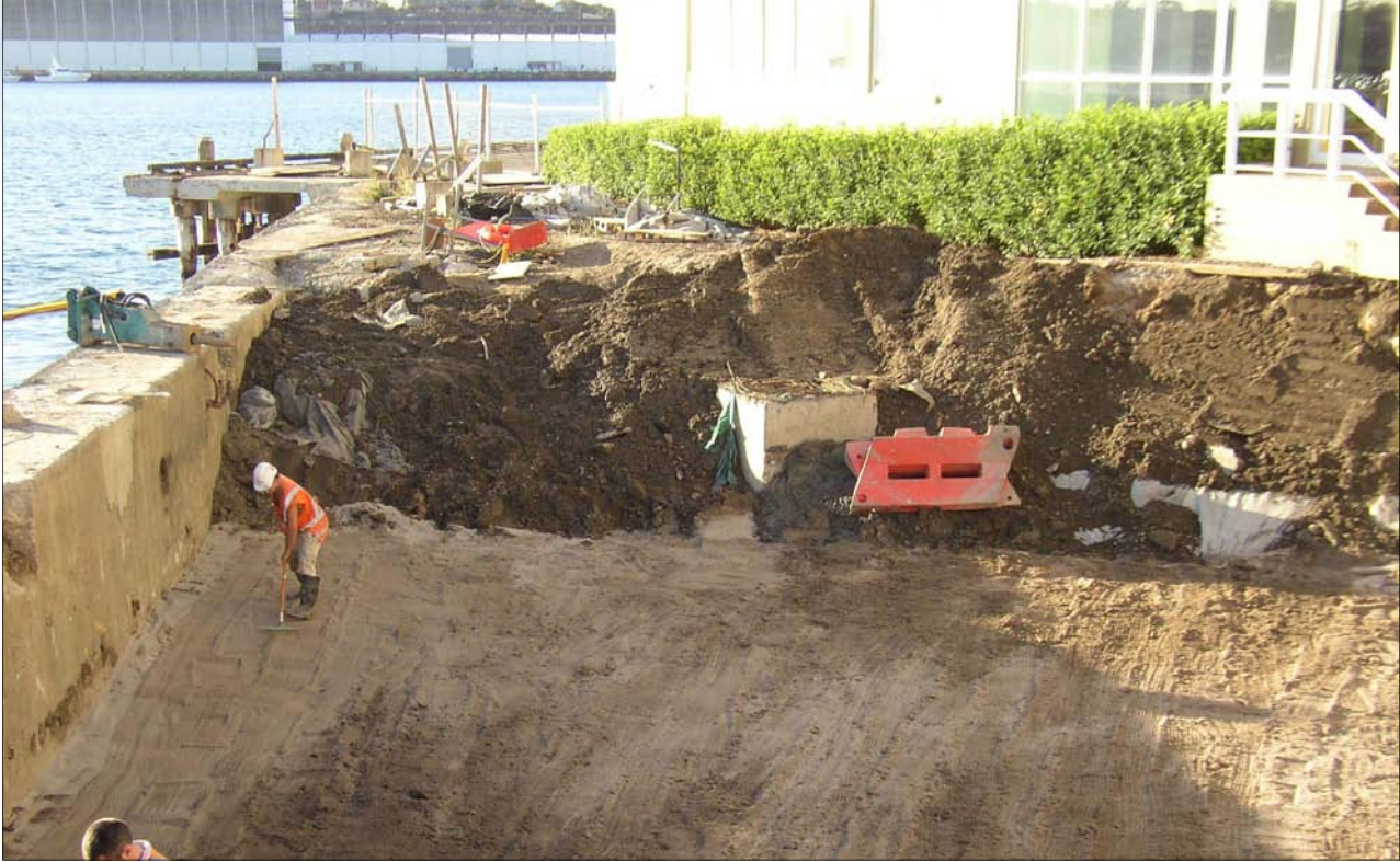
Preparing the base for the Atlantis ® Titan ® tank installation
