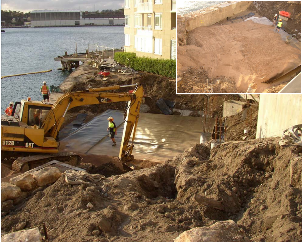
Backfilling the tank.
