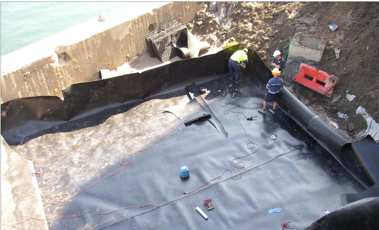
Installing the impermeable liner.
