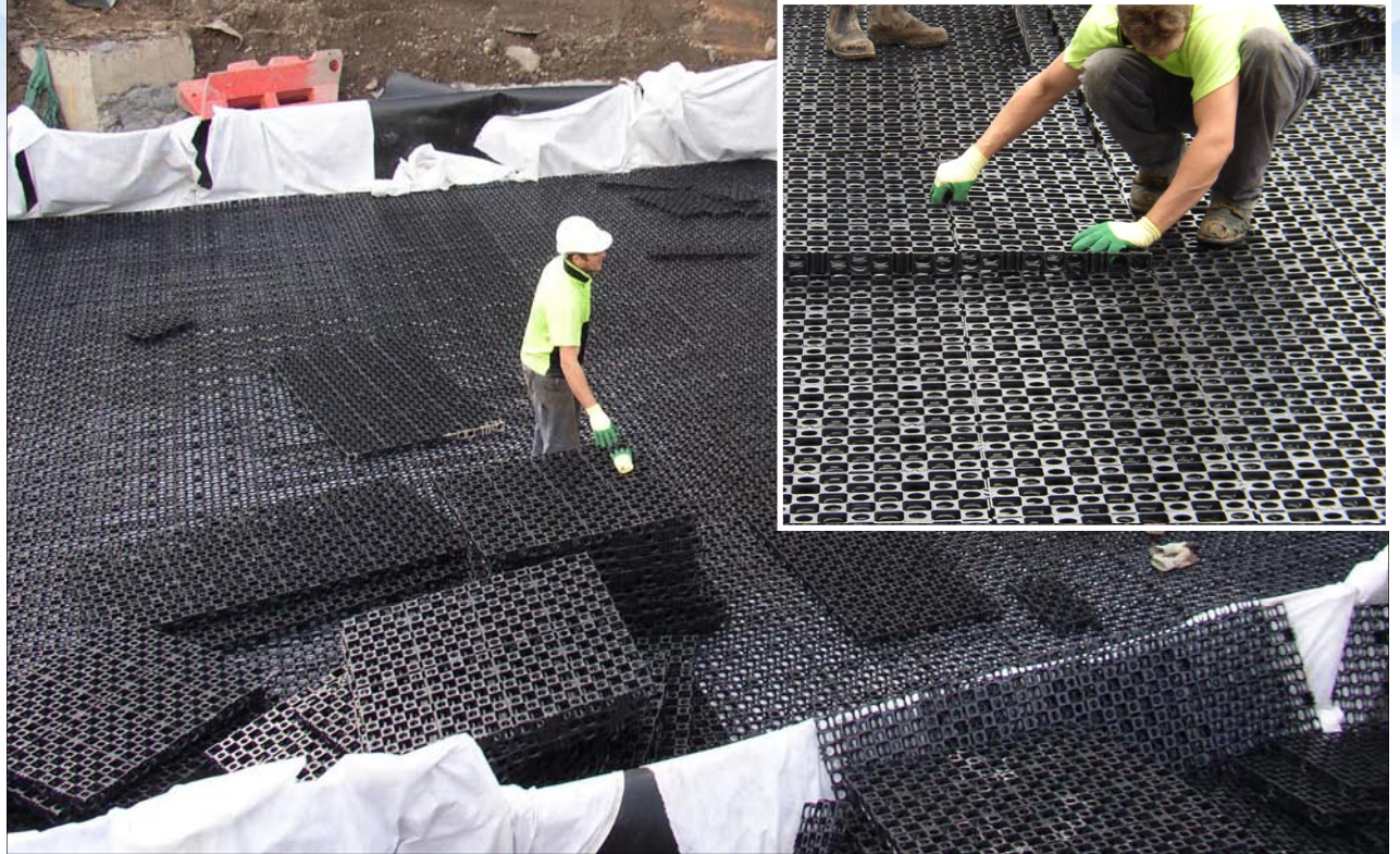
Installing the Atlantis ® Titan ® tank on top of the Geotextile fabric.
