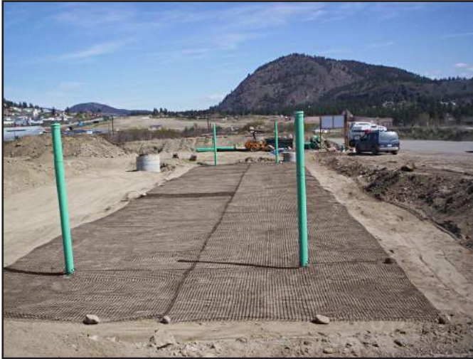
STEP 10 - Install BX-1200 geogrid.
