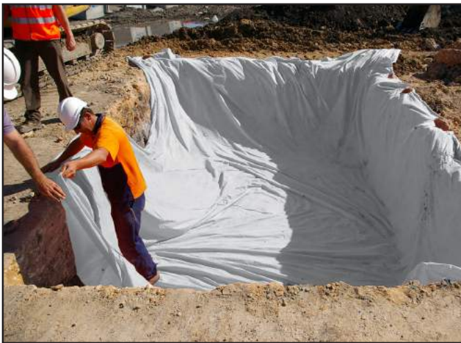
Step 3 - Lay geotextile.
