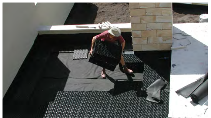
Installing Flo-Tank® modules into planter box.
