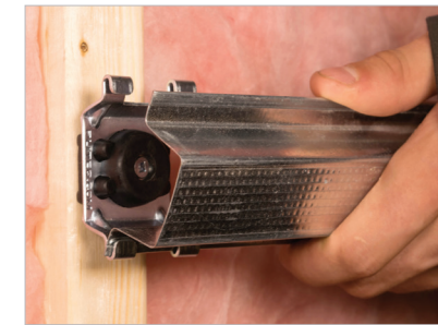
Engage standard 25 gauge drywall furring channel into either claw, then squeeze channel to engage the claw
