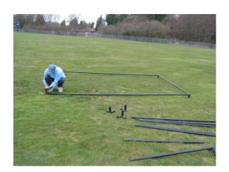
Once the top section is complete, insert a <u>female</u> pole into each of the vertical "legs" of the 3-way fittings. Be sure that the end with the small hole is at the bottom:
