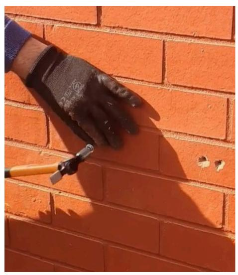
4. Secure the metal plugs using the washers then fix brackets to the wall using the screw.
