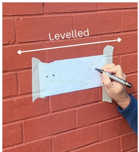
2. Drill holes exactly where you have marked using the bracket guide.
