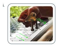
F. Then tighten the bolts with the M8 Nyluc Hex Nuts.
