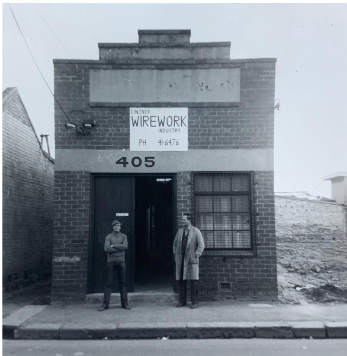
Image: Linzner father and son at the site of the original factory in 1972, located at 405 Fitzroy Street, Melbourne.
