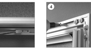
• Fix the frame to the wall through the holes in the canal.
