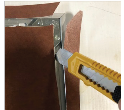
Make sure to trim off any excess banner material off the outer edge of the tacky area by inserting a box cutter knife into the channel and cutting off. This is important so that excess banner does not interfere with the CAP top rail installation.
