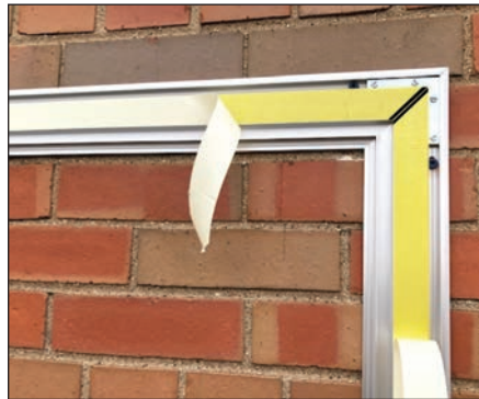
Remove masking. Tack down banner on left and right vertical BASE rails and pull tight.
