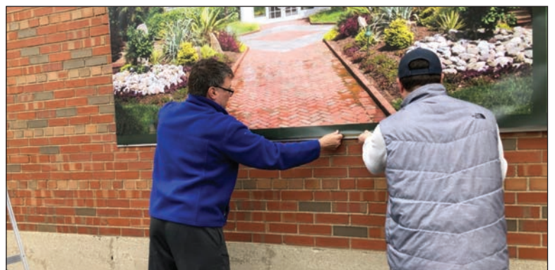
To achieve a wrinkle free banner, you must have the banner tacked to all 4 BASE rail sides in a smooth, tight, wrinkle free manner before putting the CAPS on. You can pull off the banner from the tacky tape and reposition as needed.
