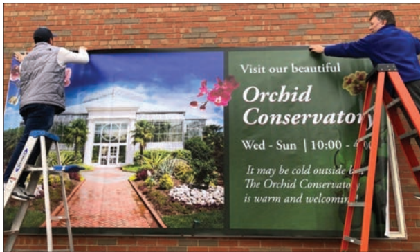
The banner must be as tight as possible, across the top and centered on the BASE rail.
