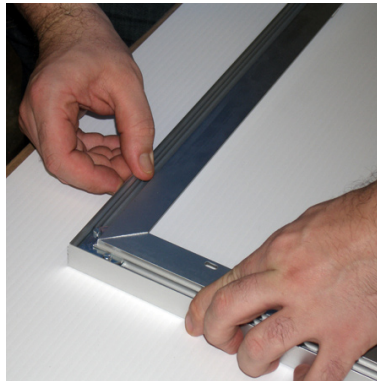
Step 5: Join Mitered Corners. The Hardware Slides Into Channel
