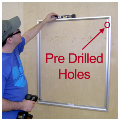
Step 8: Install Frame onto Wall with Hardware Screws Provided (Look for Pre-Drilled Holes)
