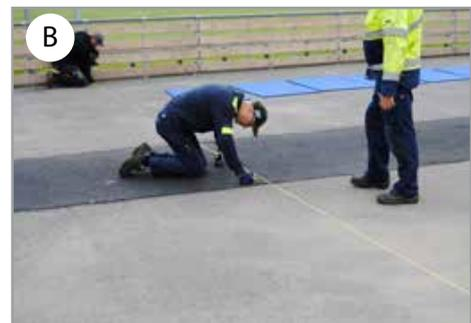
2. Lay out at least 3-4 rows of tiles or one row of pre-assembled sheets, plus the expansion strips indicated on your specific drawing so that you reach the mid-line on both the long and short sides (image C).
