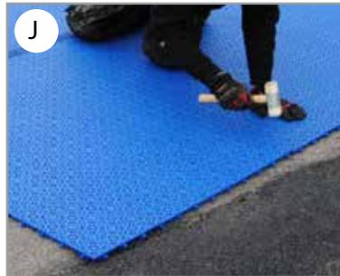
8. Continue to lay tiles according to your specific drawing for your playing area. For installation within a rink, leave the outermost row of tiles for cutting later (images G-H).
