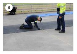
2. Lay out at least 3-4 rows of tiles or one row of pre-assembled sheets, plus the expansion strips indicated on your specific drawing so that you reach the mid-line on both the long and short sides (image C).
