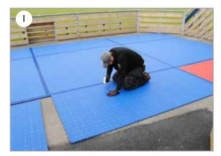
6. The rings must always be laid in the same direction, even when you are installing sheets.
