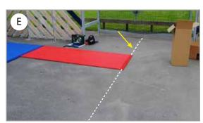
4. For installation inside a rink, leave the outermost row of tiles for cutting later and make sure that distance from the rink to the installed tiles is the same all along. Please note that the distance between tiles and rink for the short sides and the long sides need not be the same (images G and H).
