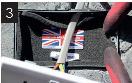
3 Insert the gasket and press firmly to attach to the box.
