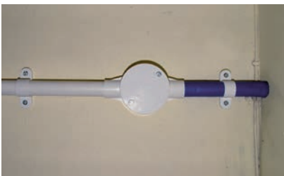
FIROBLOK CONDUIT SLEEVE FITTED INTO A 20MM BESA BOX
