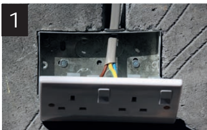
1 Insert the metal box into the wall.
