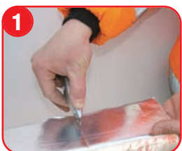
1 CUT TO DEPTH OF WALL
