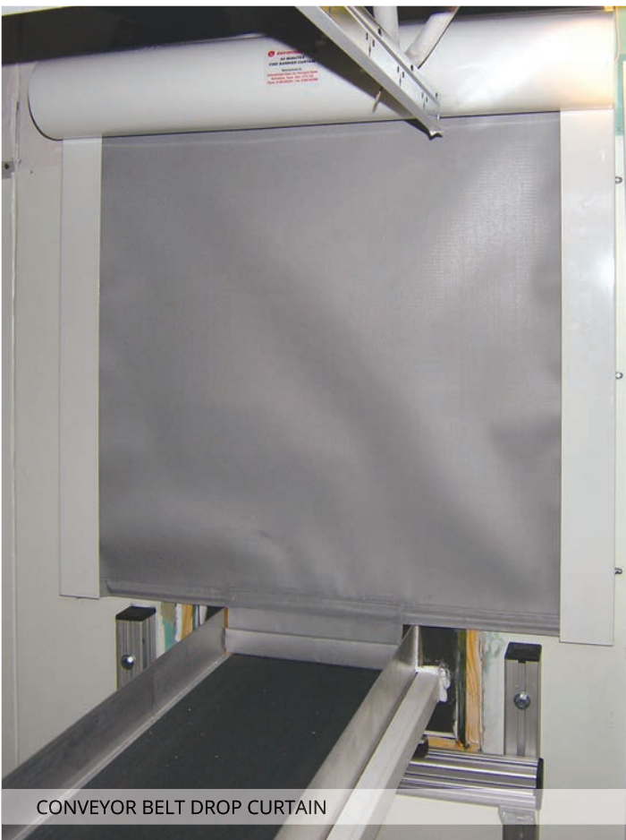
DROP CURTAIN INSTALLED AT KILWORTH HOTEL
