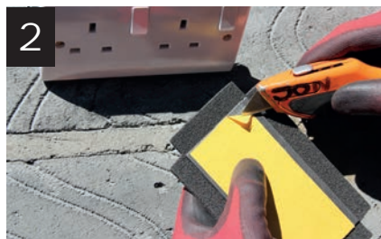
2 Peel off the protective tape.
