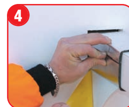
4 FIX SELF-ADHESIVE FLAP
