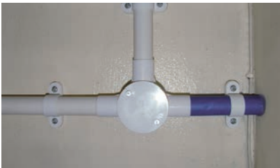
FIROBLOK CONDUIT SLEEVE FITTED INTO A 25MM BESA BOX
