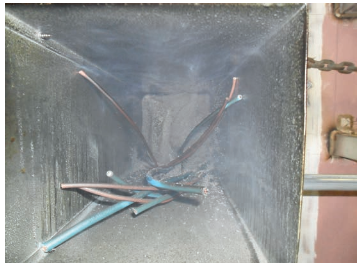
Completion of the test - trunking fully sealed
