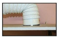
Slide the PVC or flexible PVC pipe down the unit.
