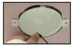
Fasten in position with supplied pins, 2 to side and 2 in the bottom holes.
