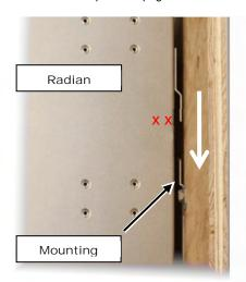
Place the Radian inverter against the wall and slide it directly over the upper lip of the mounting plate. The inverter's mounting flange should come to rest within the lip so that it hangs securely.
