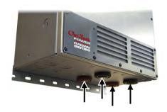
The Radian inverter has four battery cable terminals, two positive and two negative. Each terminal is a threaded hole which accepts a hex bolt (provided). Notes on assembly and cabling are shown on the next page.
