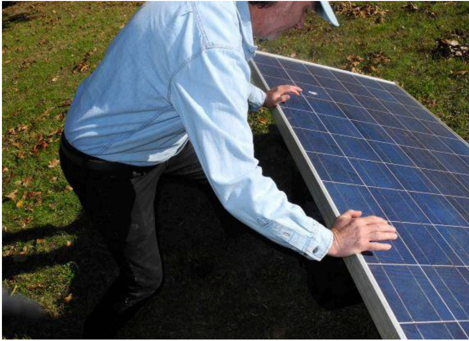
Figure 15. Worker pushing panel down into slots.
