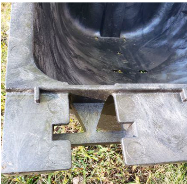
Figures 10. and 11. Close-ups of slot for sliding retainer clip
