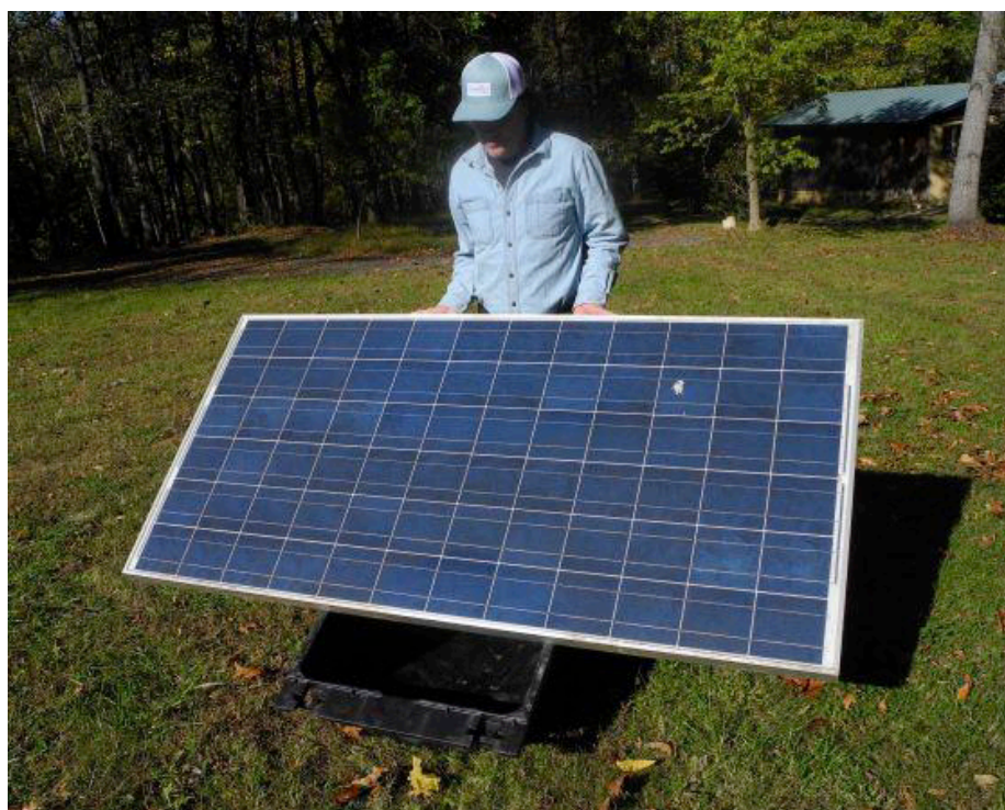
Figure 12. Worker resting panel on the PowerRack side rails ready to slide into place.
