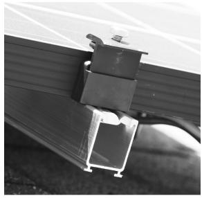
Do a final check to be sure that all installation hardware on the array is properly tightened to 12 ft. lbs.
