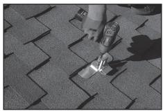
Insert the lag bolt through the sealing washer with the rubber side down and drive the bolt into the hole.
