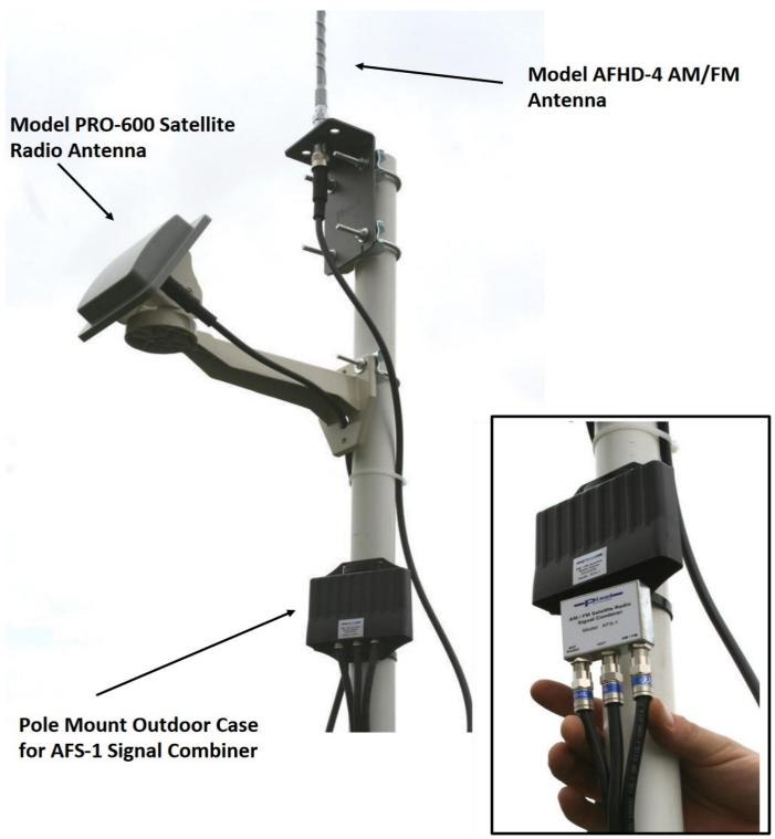
Connect All Cables Before Inserting Signal Combiner up into its case
