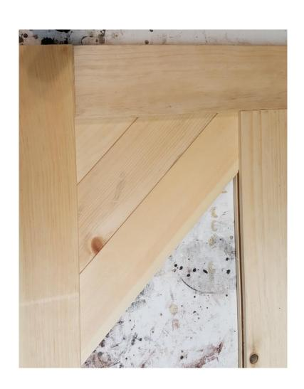
The top panels will be labelled as "TOP" on each piece. Start in the outside upper corner an install
