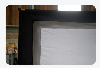
Secure screen on all four sides with Velcro frame on the inner section of bay.
