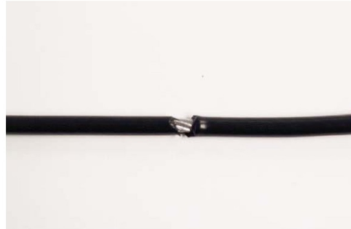
A CRACK IN THE CABLE COVER
