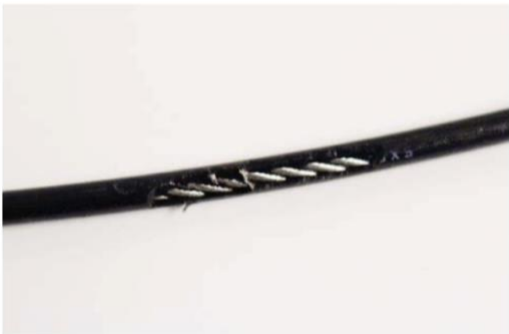
A TEAR IN THE CABLE COVER
